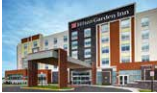
Hilton Garden Inn 50 Raritan Center Pkwy, Edison, NJ
