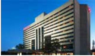
Sheraton Edison 125 Raritan Center Pkwy, Edison, NJ
